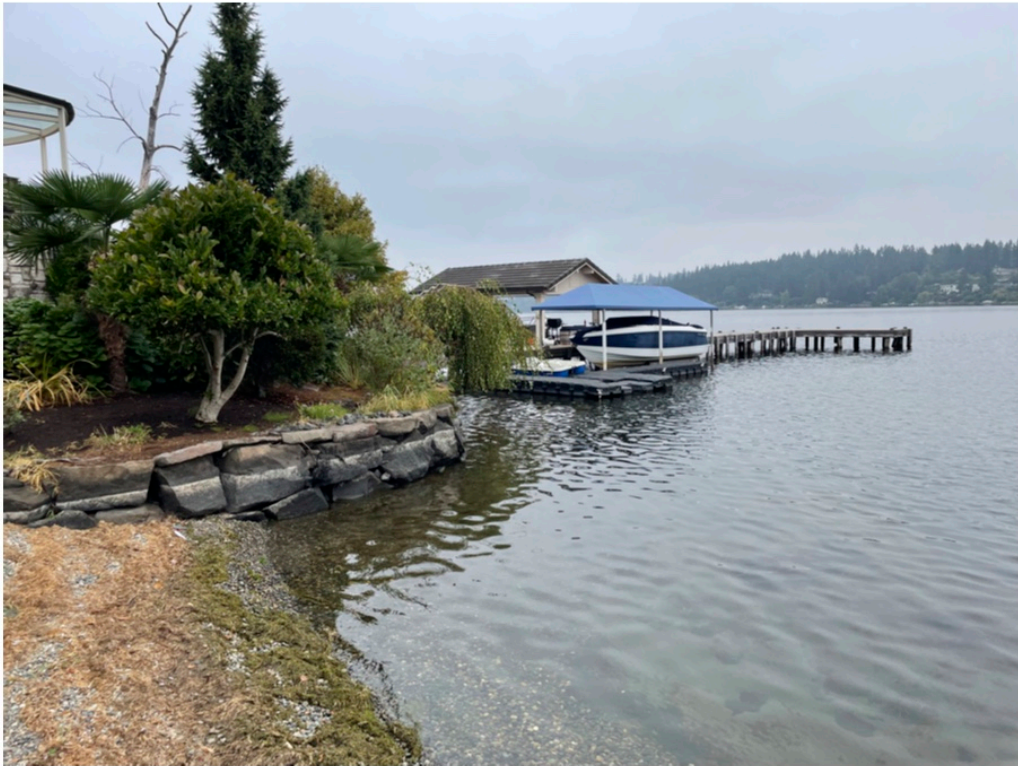
Photo 1 - Shoreline conditions where new dock will be built.
